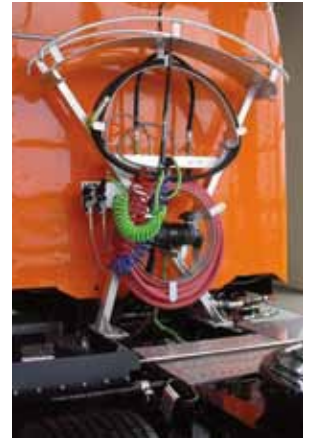
PTO/Pumps and Hose Racks
